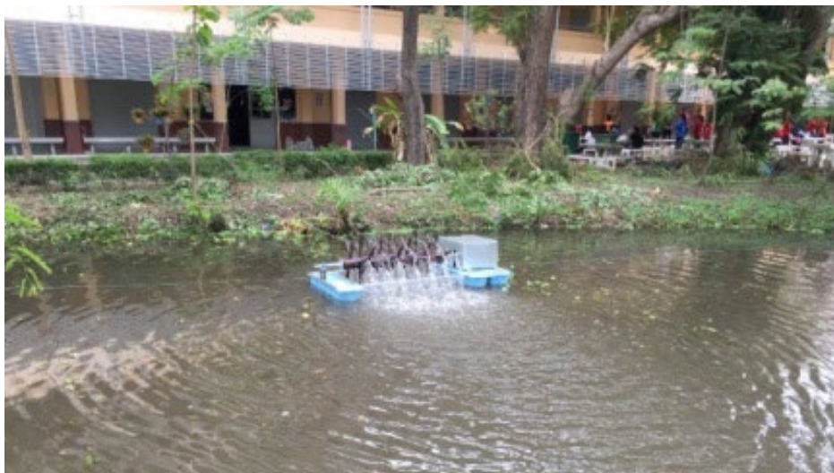
Figure 5. Equipment installation of oxygen in wastewater wells
