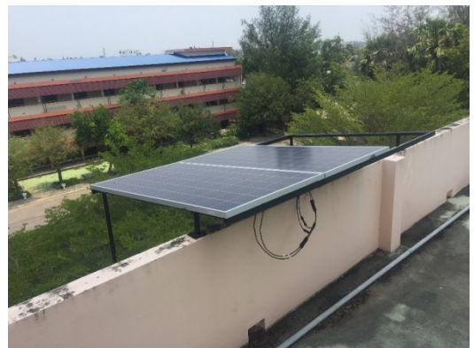
Figure 3. Installing solar cell on the roof
